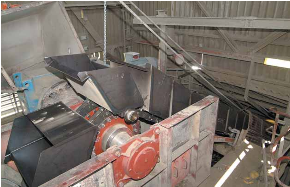
Installation of new bucket strand
