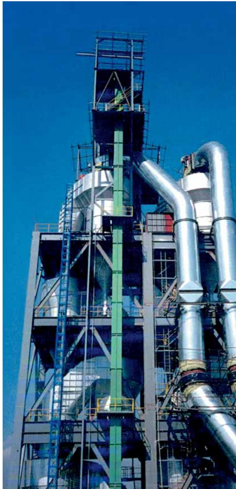
Belt Bucket Elevator for Pre-Heater Feeding
