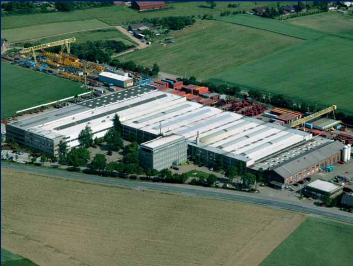
AUMUND Headquarters in Rheinberg, Germany
