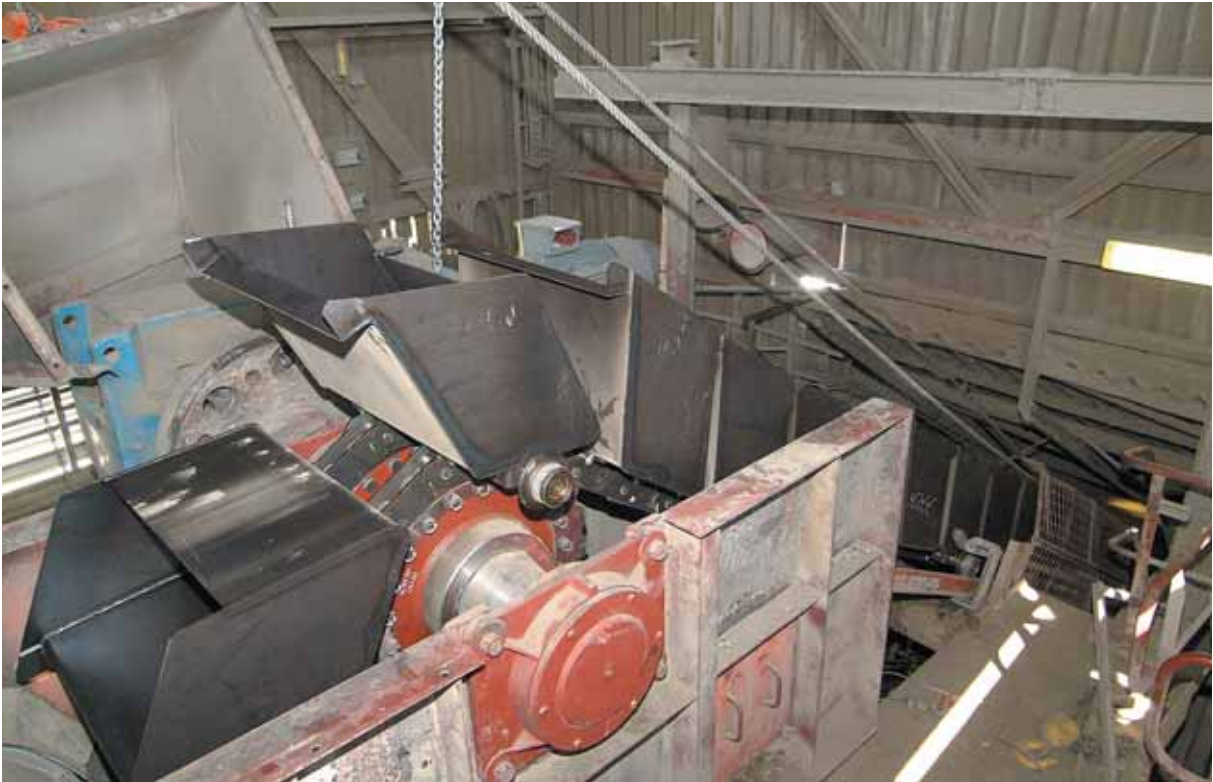
Installation of new bucket strand
