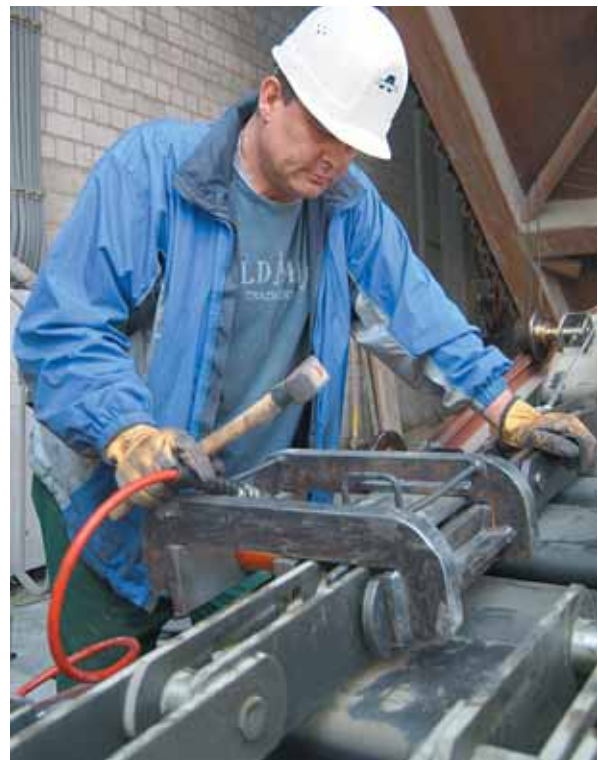
Pre-assembly of chain strands
