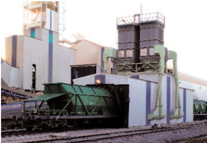
Discharge facility for Hopper Bottom Railcars receives coal for a Cement Plant including a Samson™ feeder with 80 tons holding capacity
