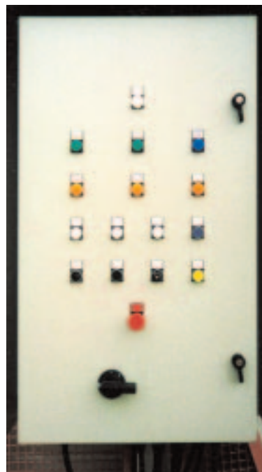
Local Cabinet with Motor Control Gear
