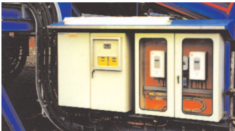
Inverter Speed Control Modules located local to the Samson™ but linked to a remote control room
